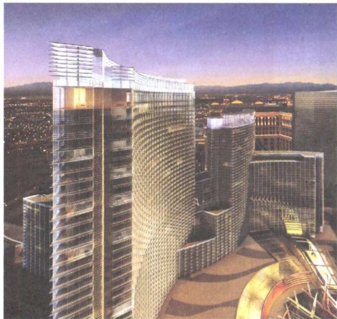
Project CityCenter by MGM Mirage will be the largest LEED-certified development of its kind in the U.S.
